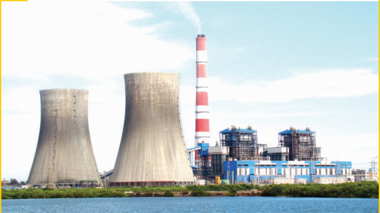
Panoramic View of the Plant
