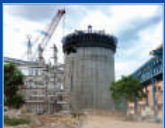
FGD & Additional Chimney Construction
