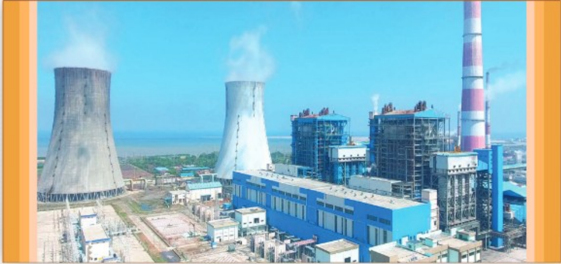
Panoramic View of the Plant
